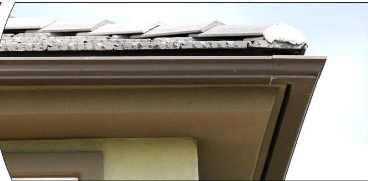
Eaves are the underneath part of the roof that extends beyond the home's outer wall to the roof's edge.
